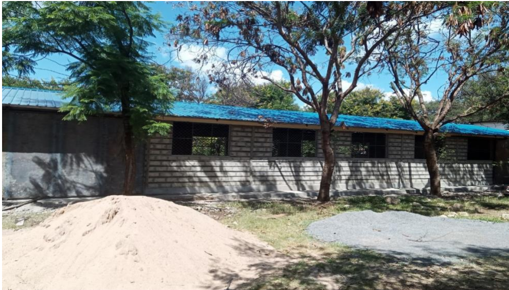
Roofed section of the rehabilitated St Joseph Polytechnic's Production Department
