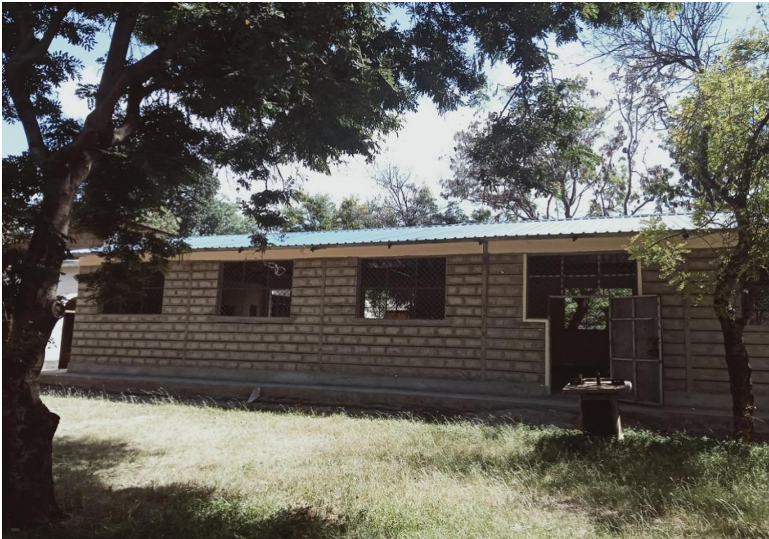
A section of the completed workshop from the front side.
