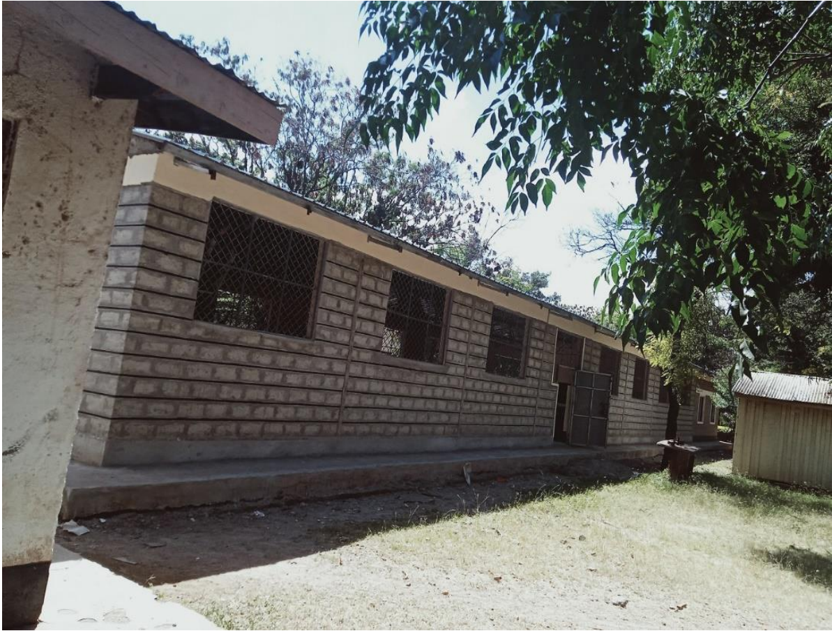
A section of the completed workshop from the back side.
