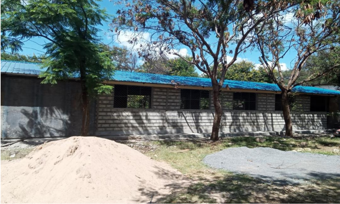
Roofed section of the rehabilitated workshop
